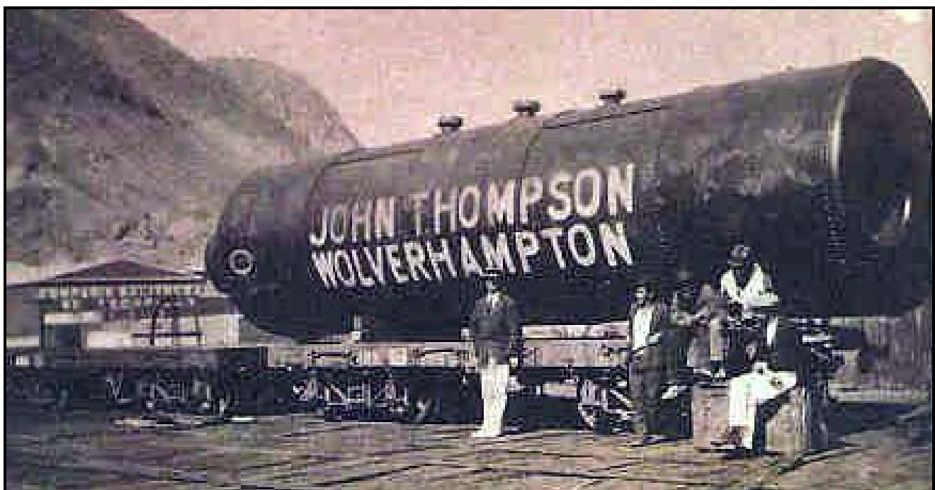
A John Thompson boiler being transported across Chile in the 1920s
